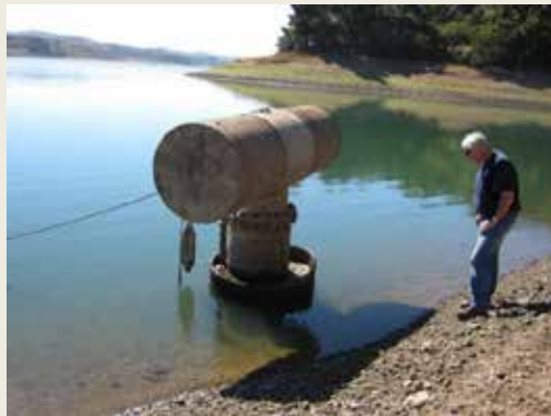
Figure 3 - Upper Intake at Crystal Springs Reservoir, August 2007
