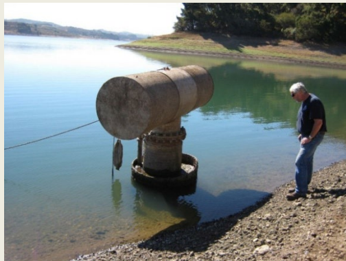
Figure 3 - Upper Intake at Crystal Springs Reservoir, August 2007
