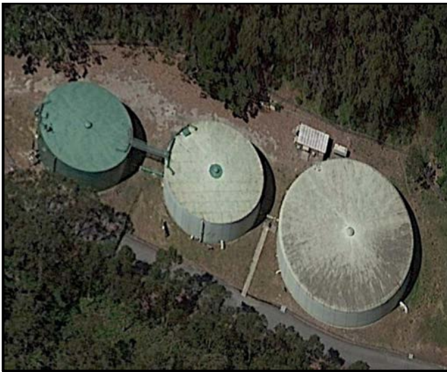
Future Project Replacement of Treated Water Storage Tanks
