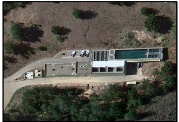
Future Project Nunes Water Treatment Plant Improvements
