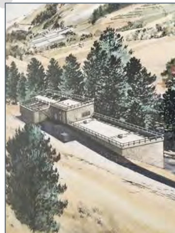
Nunes Water Treatment Plant
