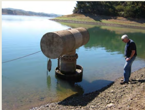
Figure 3 - Upper Intake at Crystal Springs Reservoir, August 2007
