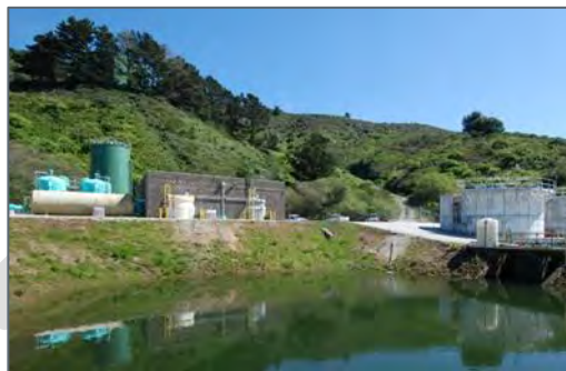
Denniston Water Treatment Plant
