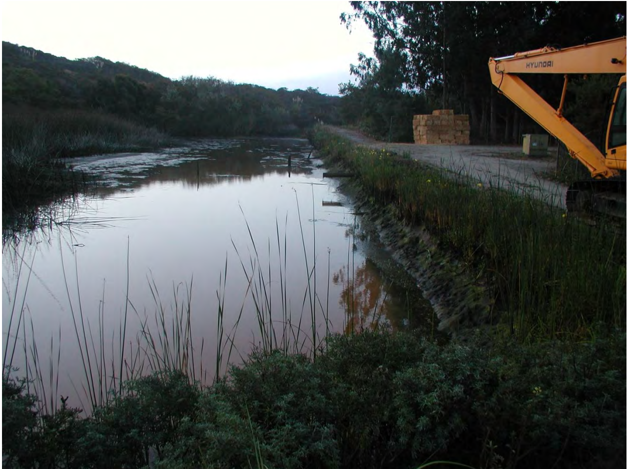
Hay bales are ready to place. Water is drawn down.
