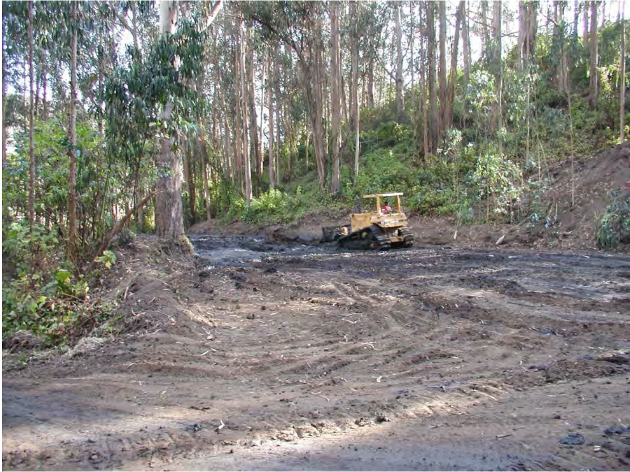
Spoils site is maintained by concentrating sediment and has containment berm.
