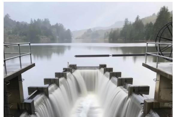
Pilarcitos Reservoir Spillway
