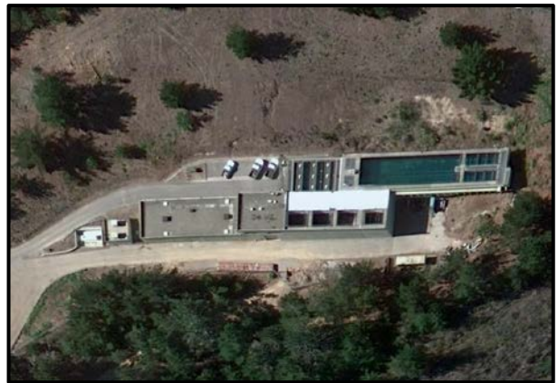
Future Project Nunes Water Treatment Plant Improvements
