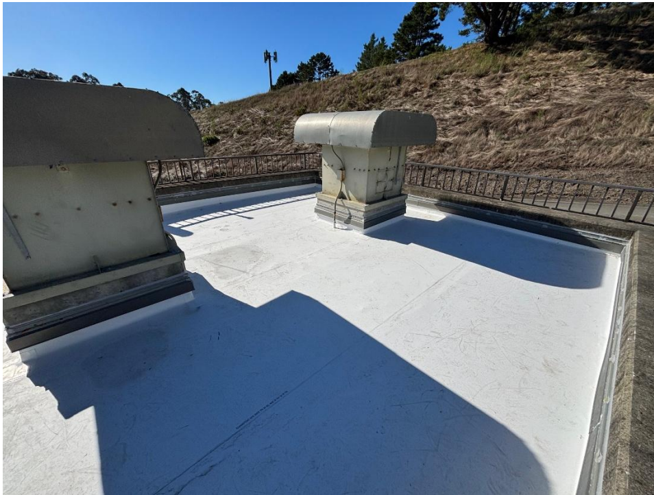
Nunes Generator Roof Completed October 2025
