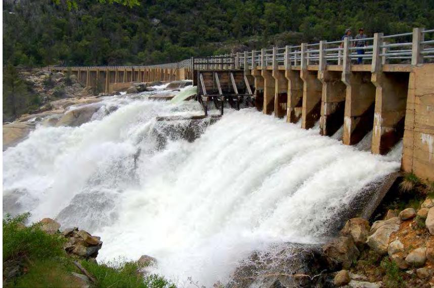
**Lake Eleanor** – The dam at Lake Eleanor is 1,260 feet long, has a maximum height of 61 feet and creates a 27,500 acre-feet reservoir in the western-most part of Yosemite National Park. The dam was completed in 1918 and was the first reservoir in the Hetch Hetchy system. The dam is designed to make use of the spillway during snowmelt runoff (B. McGurk).
