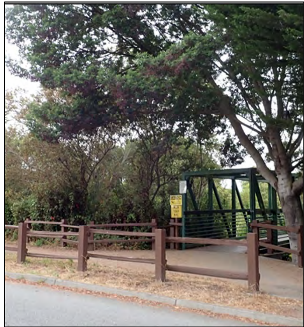
Photo 7c: Southwest view into Bridge Entrance from San Mateo Road
