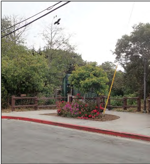
Photo 7b: Northeast view into Bridge Entrance from Pilarcitos Avenue.
