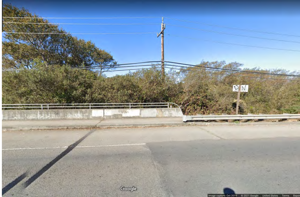
Figure 8. View from SR-1 looking west at Pilarcitos Creek bridge.
