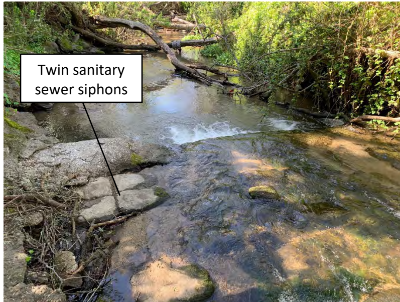
Figure 5 – Exposed twin sanitary sewer siphons in Pilarcitos Creek, facing west.
