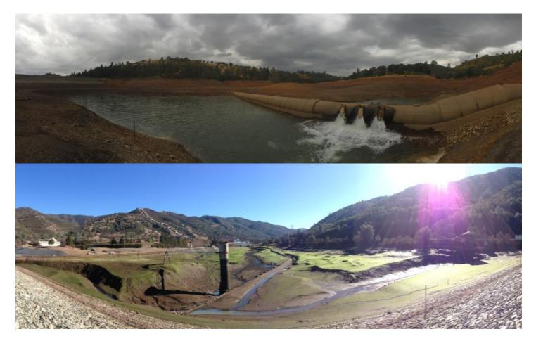
Priest and Moccasin Reservoirs have bypass capabilities. Under normal operations, neither bypass is in use. One or both can be used with no impact on delivery capacity in case of water quality or operational concerns.
