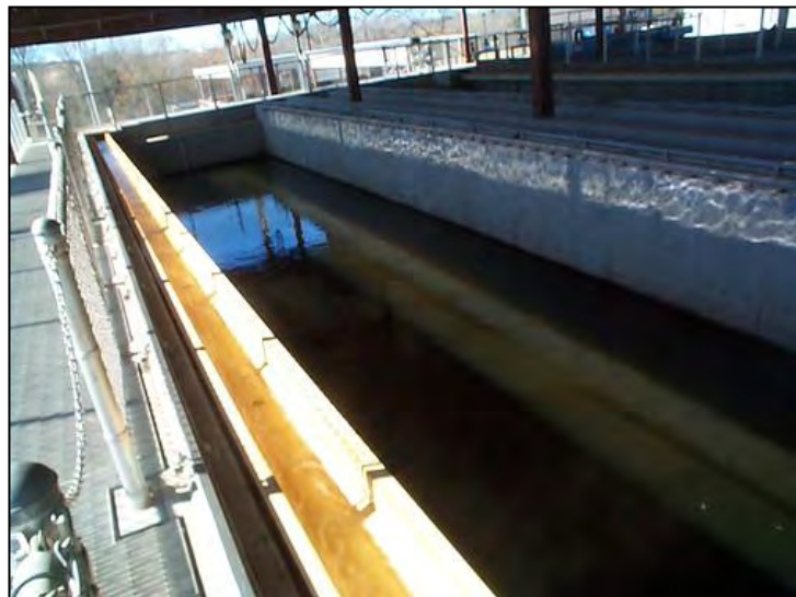
Figure 4.2 Typical Filter Bed
