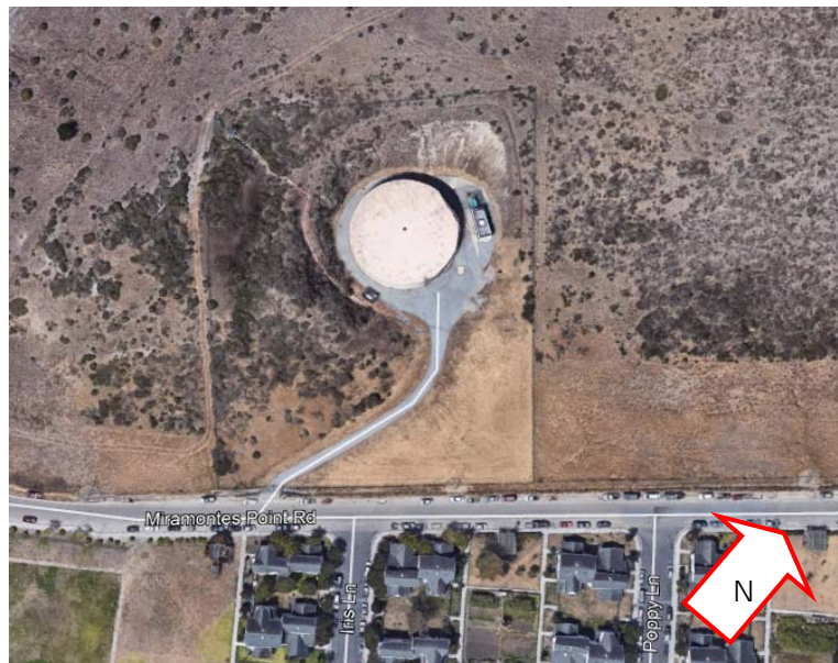
Figure 2: Alves Tank Site Photo (Source: Google Earth)
