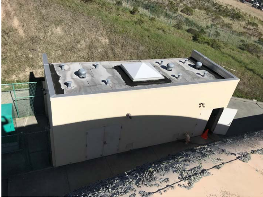
Photo 9: Pump House Building
