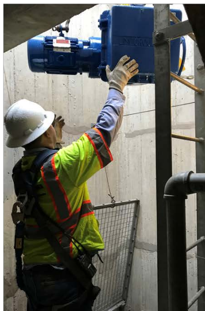
The Hetch Hetchy Water and Power Mechanics and Labor Crew lower a replacement actuator for one of the eight O'Shaughnessy Dam face release valves.
