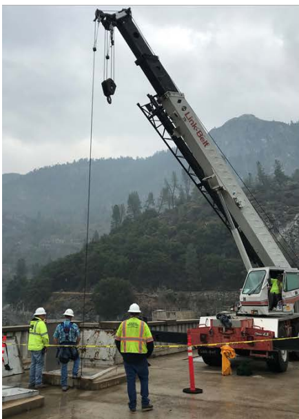
The Hetch Hetchy Water and Power Mechanics and Labor Crew lower a replacement actuator for one of the eight O'Shaughnessy Dam face release valves.
