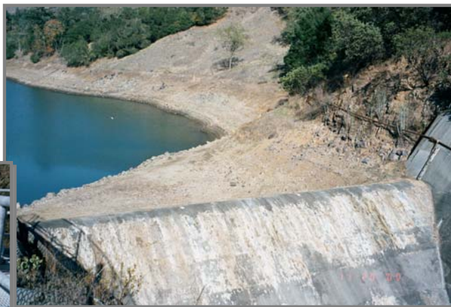
View of Kimball Dam and the proposed location of the inflatable dam
