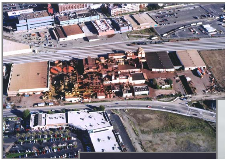
Prior to Demolition
