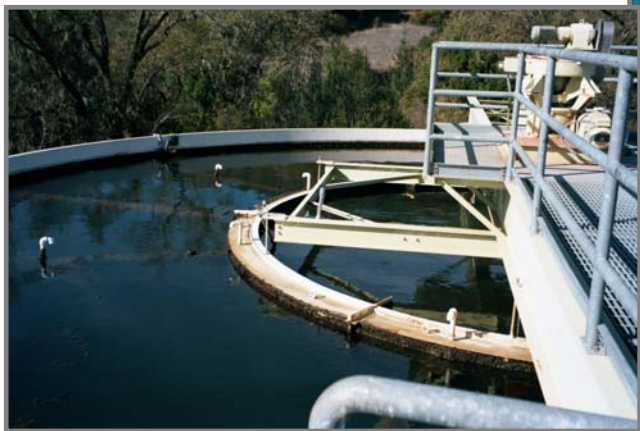
View of the primary clarifier to be modified as part of the project
