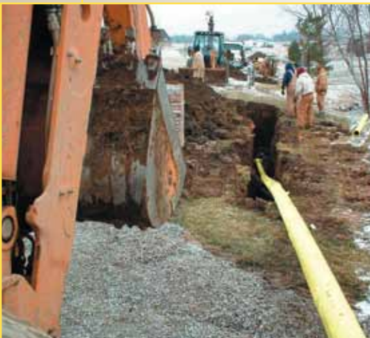
Yelomine IB trenchless installation
