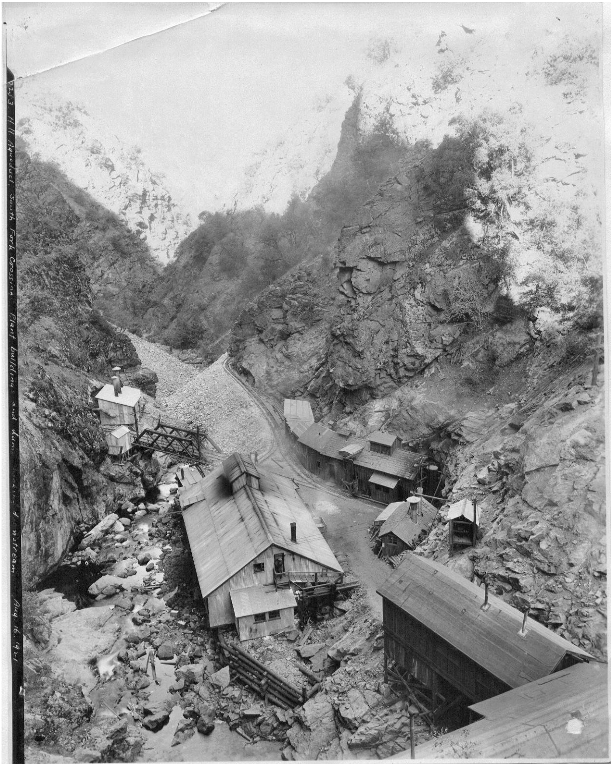
The South Fork Crossing Camp on the South Fork of the Tuolumne River was one of the access points for the boring of Mountain Tunnel. The camp was riddled by rockfall due to the steep terrain. A pipe was initially installed to span the canyon, however due to the amount of damage caused by rockfall on the pipe, a tunnel was later bored under the river.
