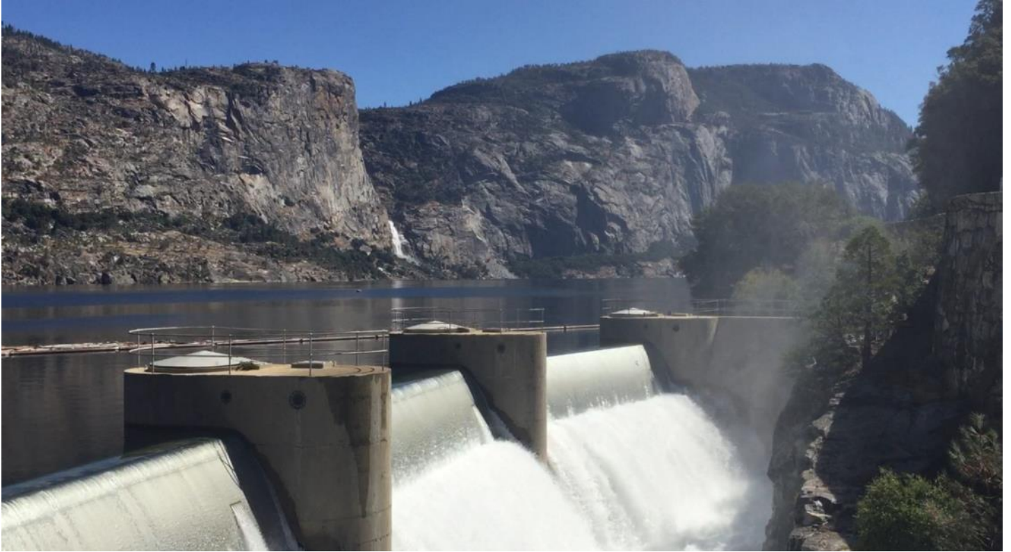
Spill from the Hetch Hetchy drumgates at the end of runoff, July 28 2017.
