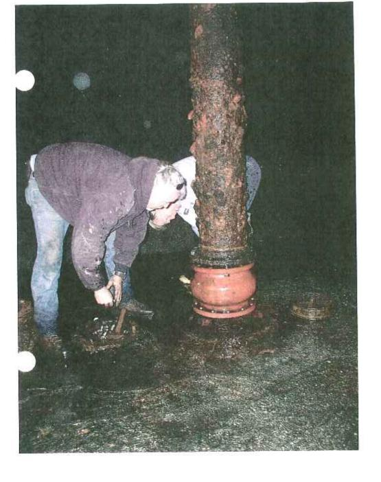
Temporary foot valve for 60 hp high lift pump at Denniston.
