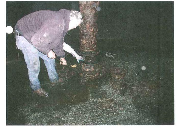
Removing original failed foot valve at Denniston.
