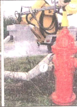
Flow Test Hydrants
