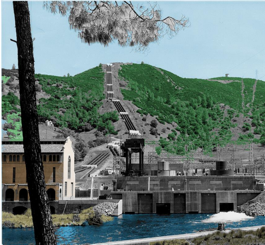
Moccasin Powerhouse and Penstocks
