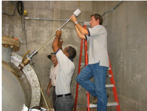
Figure 4: Installation of Reference Meter
