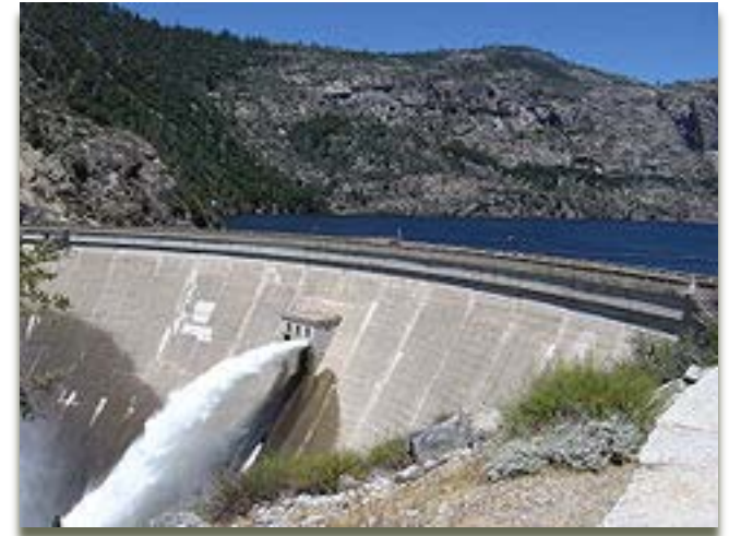
O'Shaughnessy Dam @ Hetch Hetchy Reservoir
