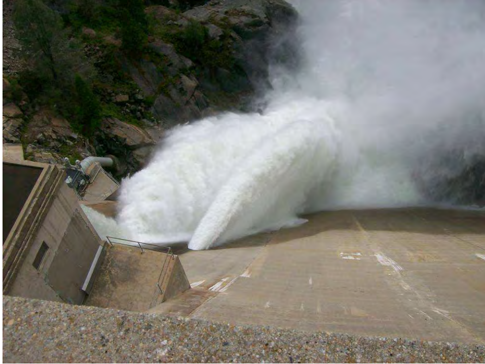
O'Shaughnessy Dam – Large releases of 8,100 cfs were made from Hetch Hetchy at the end of May as part of the Upper Tuolumne River Ecosystem Project (K. McRorie)
