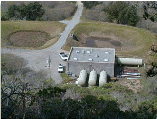
Denniston Water Treatment Plant
