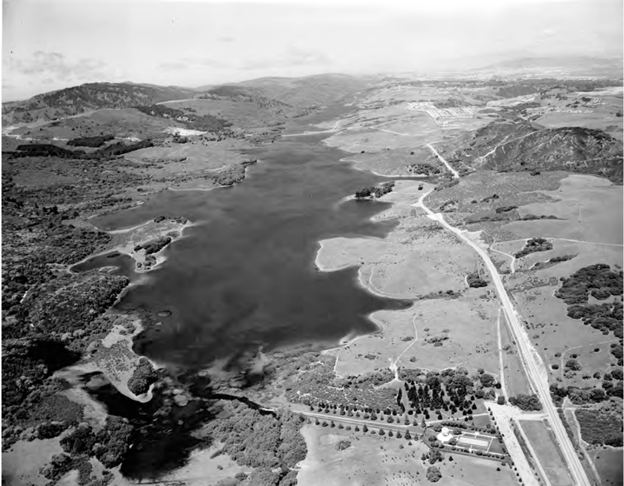
View of Crystal Springs Reservoir (Upper and Lower) looking north, April 1960. The Pulgas Water Temple and water conveyance channel to Upper Crystal Springs are in the foreground. Lower Crystal Springs is seen in the background beyond the CA Hwy 92 traverse atop Upper Crystal Springs Dam (c. 1877). Note Hwy 280 is still on the drawing board and not in sight.
