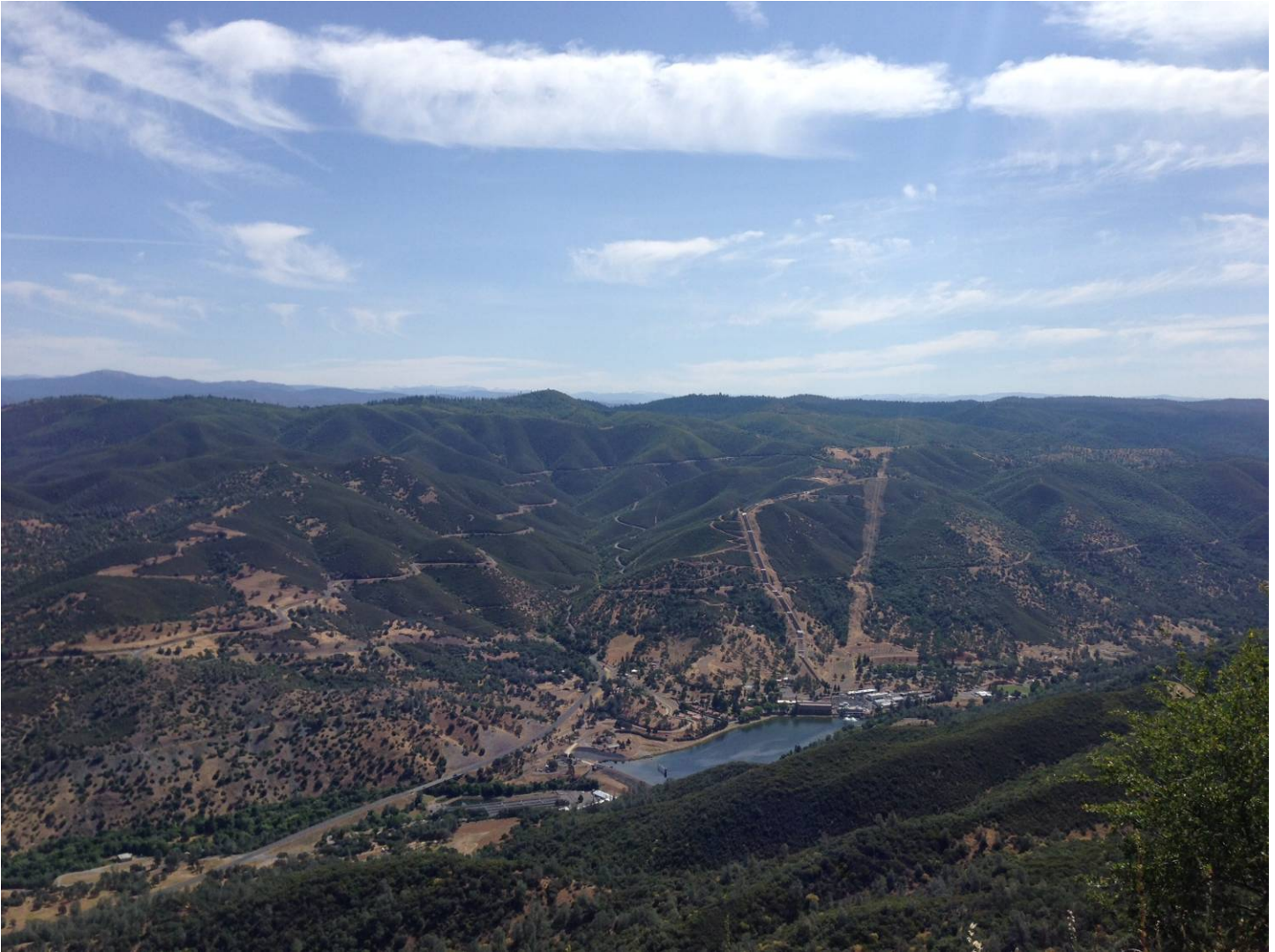
Moccasin Reservoir and Powerhouse, as seen from Moccasin Peak
