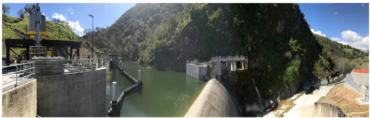
Alameda Creek Diversion upgrades include fish screens on the tunnel intake and a fish ladder.
