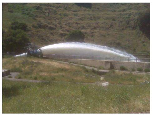
**Calaveras Dam** – A large "cone" valve releases 150 cfs of water from Calaveras Reservoir in order to control reservoir elevation. The valve, affectionately known as "Big Blue", can release up to 800 cfs (A. Dhakal).
