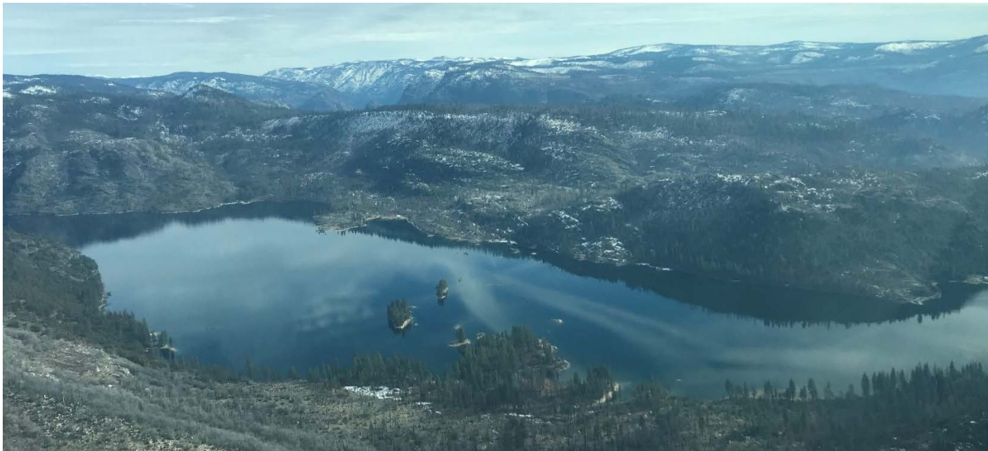
Lake Eleanor Reservoir. Elevation 4655 ft with a capacity of 21,500 acre-feet. As seen from the air January 25, 2020
