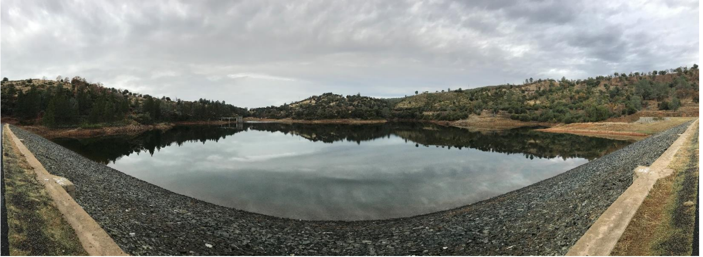
Priest Reservoir as seen from the dam. Priest is a regulating reservoir for Kirkwood Powerhouse and Moccasin Powerhouse. Storage capacity is approximately 2000 acre-feet.
