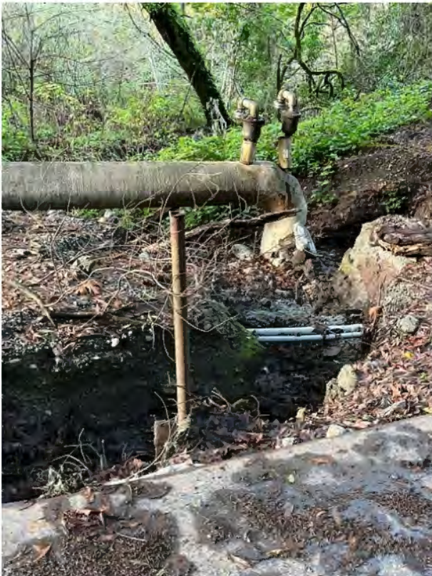
Damaged Culvert
